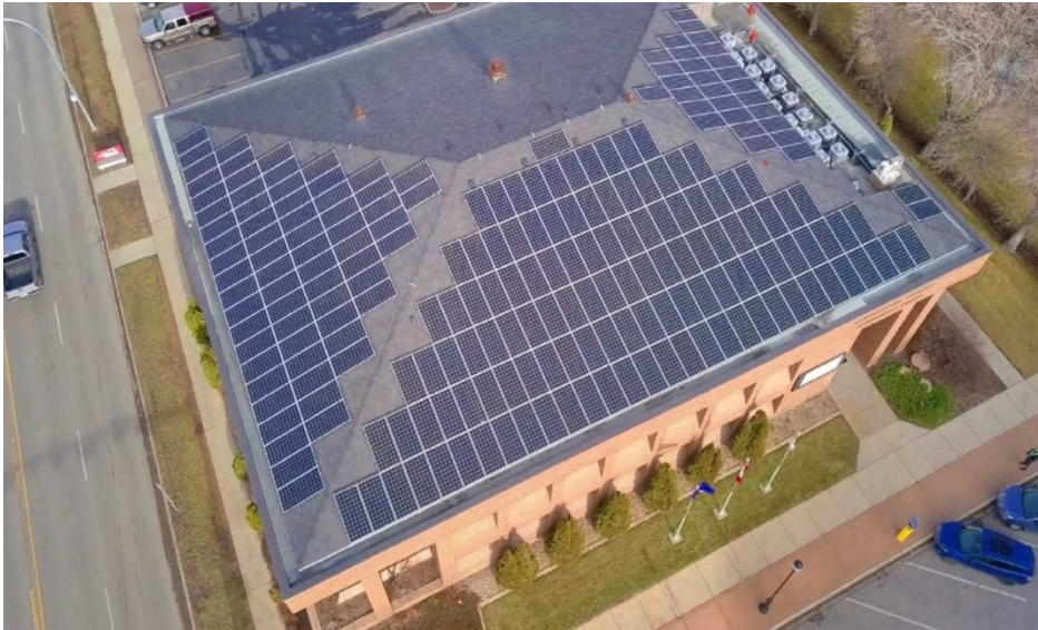
Figure 5. Auto-generating photovoltaic system
