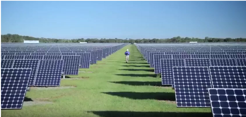
Figure 4. Solar power park
